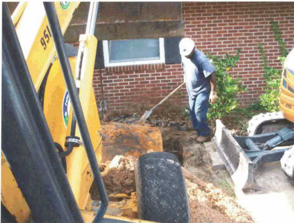
Picture 2: UST 1283Dove being removed from the excavation.
